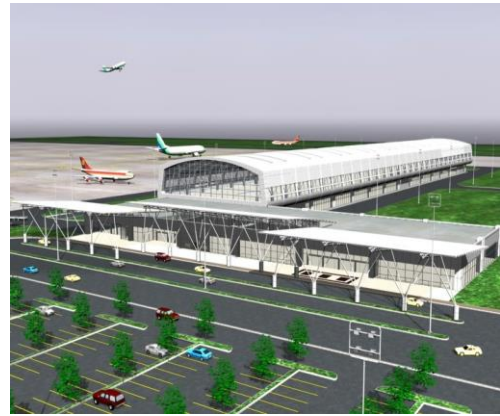
Picture 14: Bird eye view of Terminal 3 Phase I. Note the semi arch roof structure of the airside building formed by the steel frame. (Source: tritunggalprima.com )
