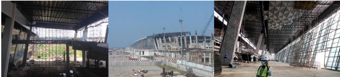
Picture 19: Terminal 3 Ultimate under construction. (Source: left - kompas.com; centre - Wikipedia; right - thepresidentpostindonesia.com)
