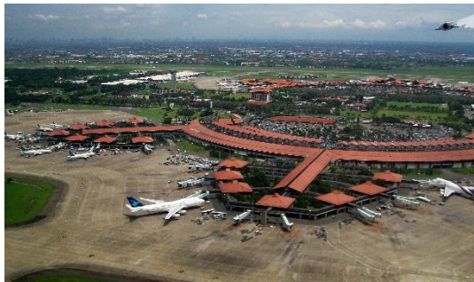
Picture 2: Aerial View of Terminal 1 and 2 (Source: Wikipedia)
