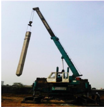
Gambar 3 Lifting pile
